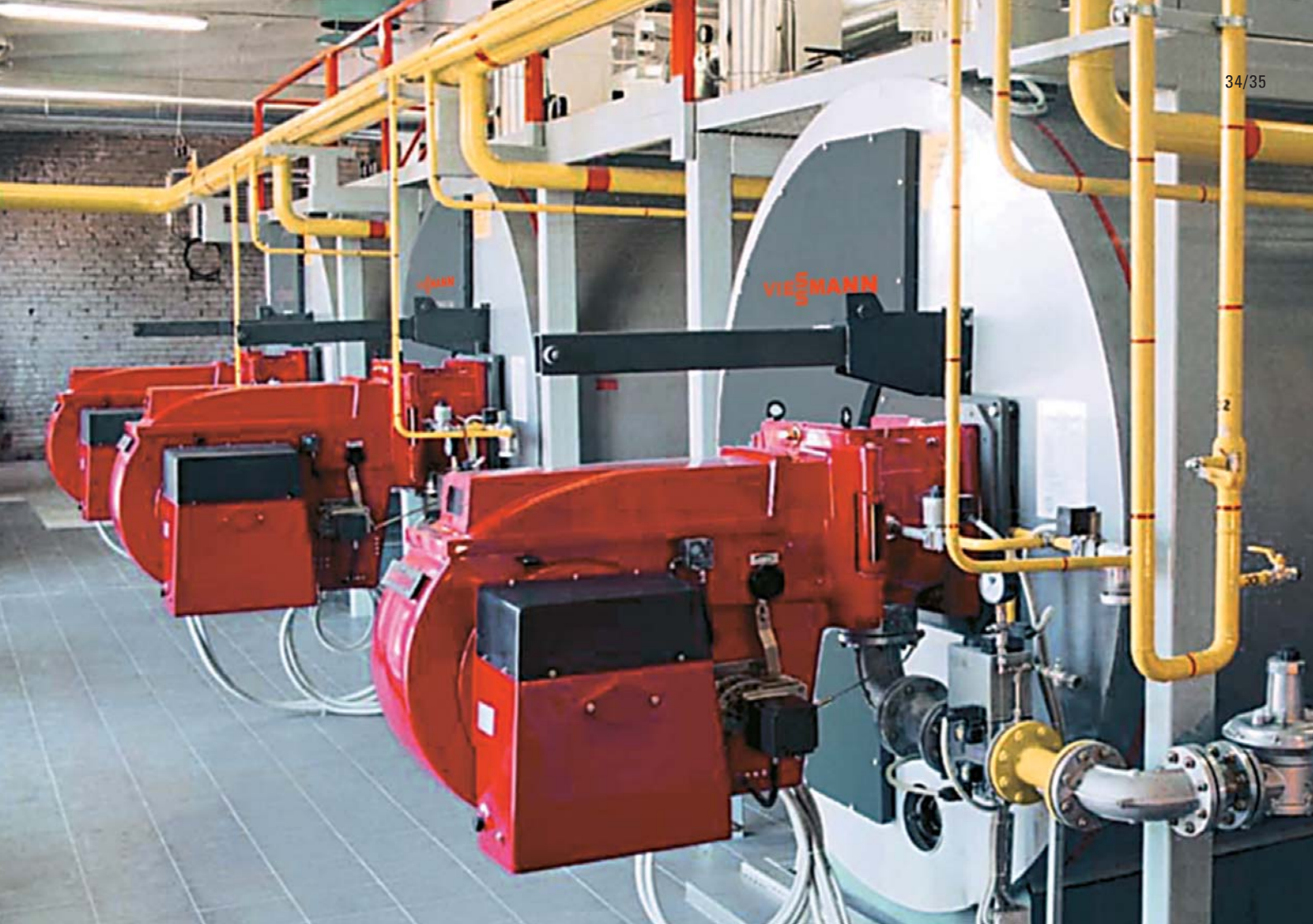
Vitomax 300-LT, low temperature hot water boiler
